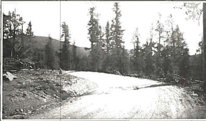
Looking south around switchback at station 90 west.
