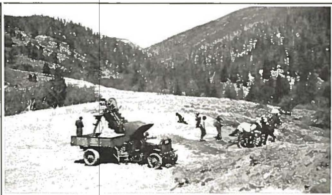
Loading surfacing in pit at Station 470 West.
