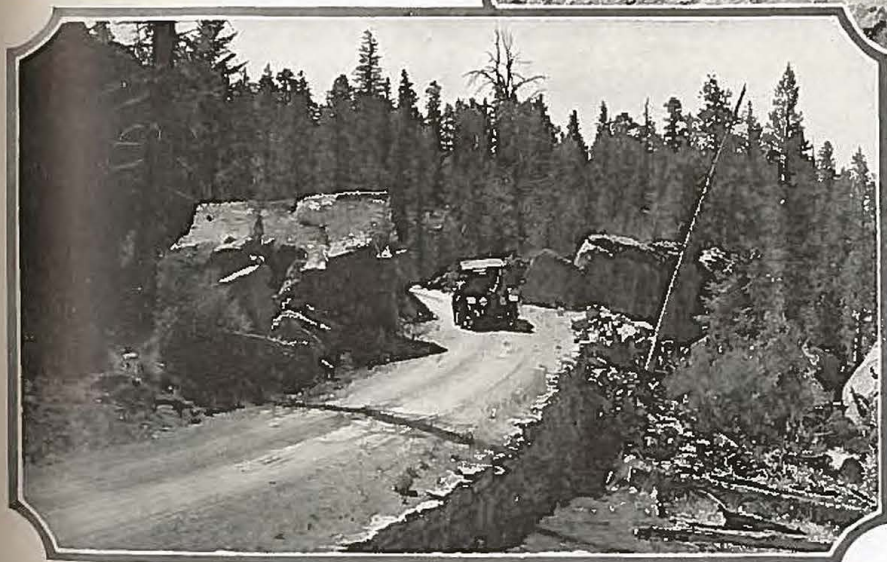
View of completed forest road on Rabbit Ear Pass in Grand County.
