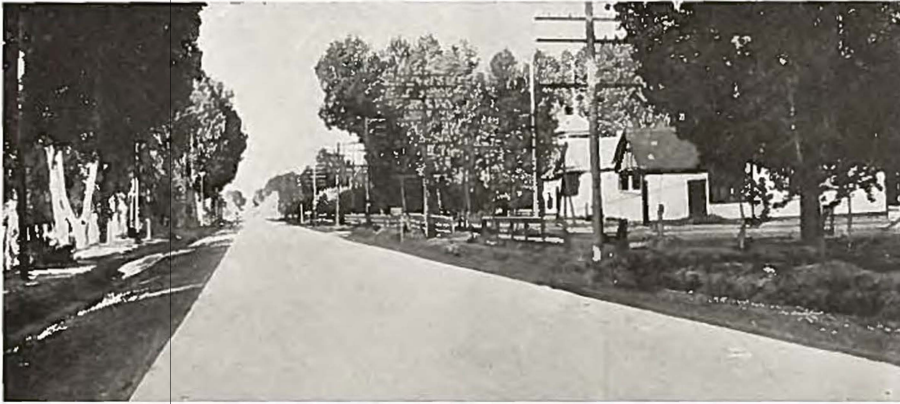
A fine stretch of concrete paving cast of Grand Junction in Mesa county.
