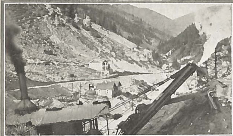
A view showing old road and new road with steam shovel in action near Red Cliff. (Lower left) Steam shovel moving up grade from Gilman. (Right) Perpendicular wall at Lover's Leap, where sixteen feet of solid rock was blasted away to make road passage.
