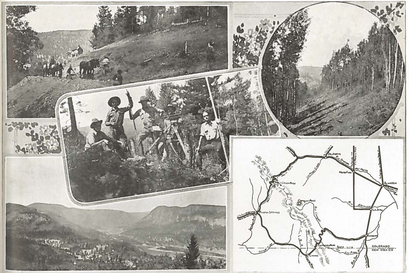
Showing State Highway work in progress on Cumbres Pass in Conejos County. Upper left: Conejos County forces removing difficult boulder material. (Circle) Clearing for new road. (Center) Engineering party, left to right, William Blackstone, George Fitzmorris, Robert Wallace, H. O. Lemon, Walter Wilson and W. M. McLeod. (Lower left) View from Station 194, with Conejos River in the distance. (Lower right) Map showing route of new road from Antonito to Pagosa Springs.
