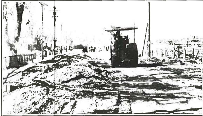
Steam roller at work on sub-grade.
