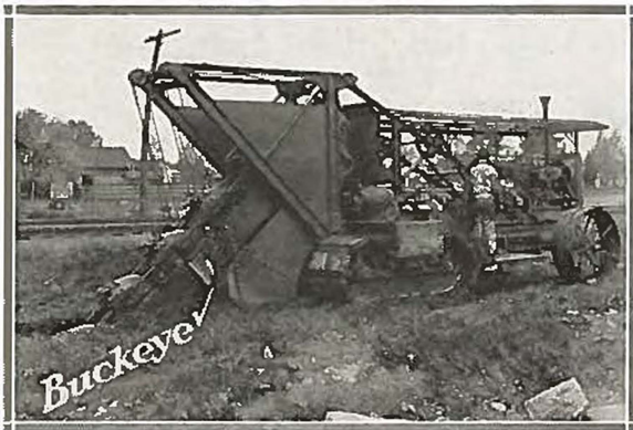
The Buckeye Chain and Bucket Excavators
