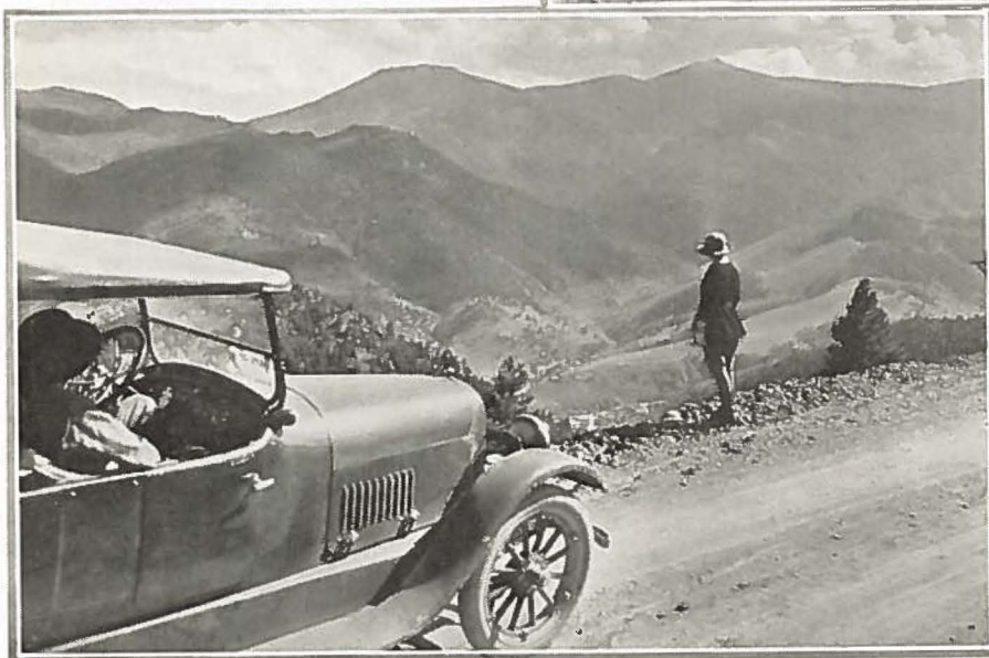
Two views of new Virginia Canon road recently completed by State Highway forces. Lower picture shows Idaho Springs in the valley below and Mt. Evans in the Distance.
