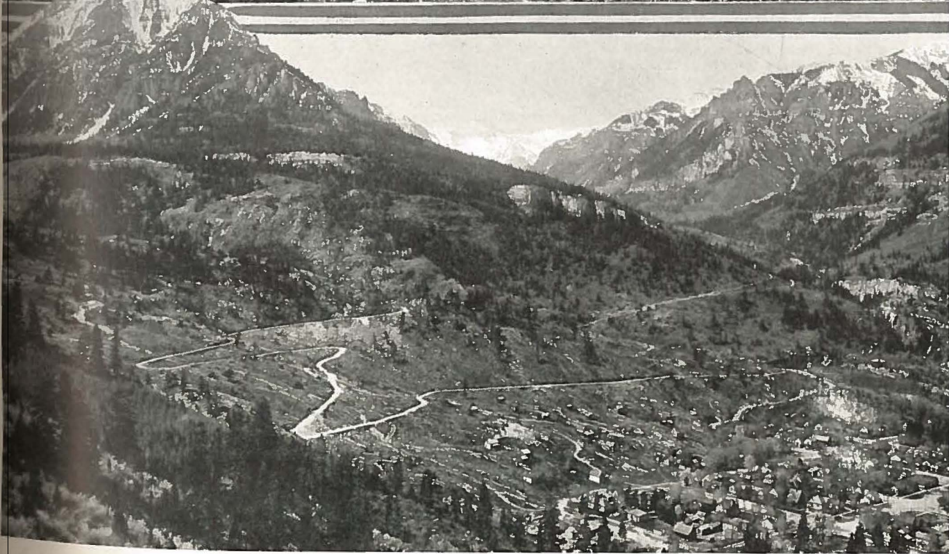
The Ouray-Silverton Road is one of the most picturesque in Colorado. Upper picture shows part of the heavy construction, a double hairpin loop, and the lower photograph a part of the pioneer mining town of Silverton.
