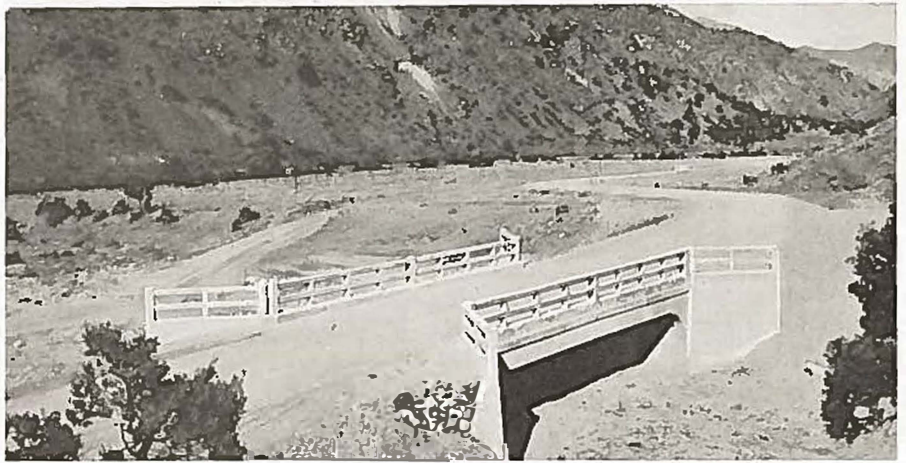
A fine example of concrete bridge construction in Chaffee county. Built with Federal Aid funds.
