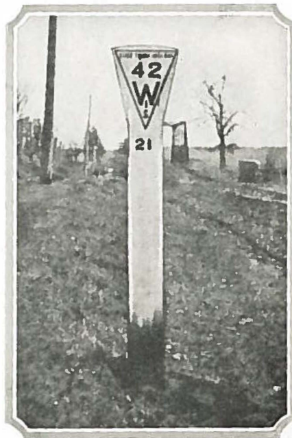
Fig. 2. The standard Trunk Highway mile post, showing within the triangle the Trunk Highway number and below the mile number. (C. 406.)
