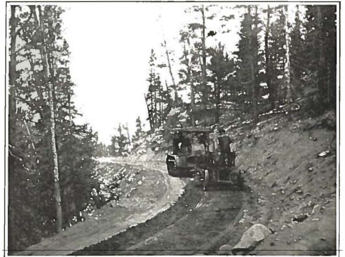
Fifteen-ton Holt tractor and Adams Giant Road King used in grading.
