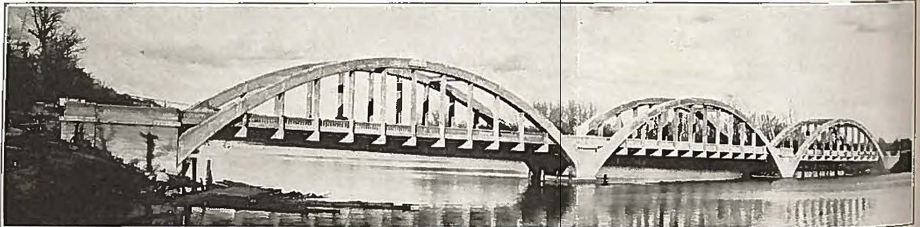
Marsh Rainbow Arch Bridge. This type of bridge will be constructed over the Platte River, at Ft. Morgan, Colo. 1190-foot spans; total length 1060 feet; longest bridge in the state.
