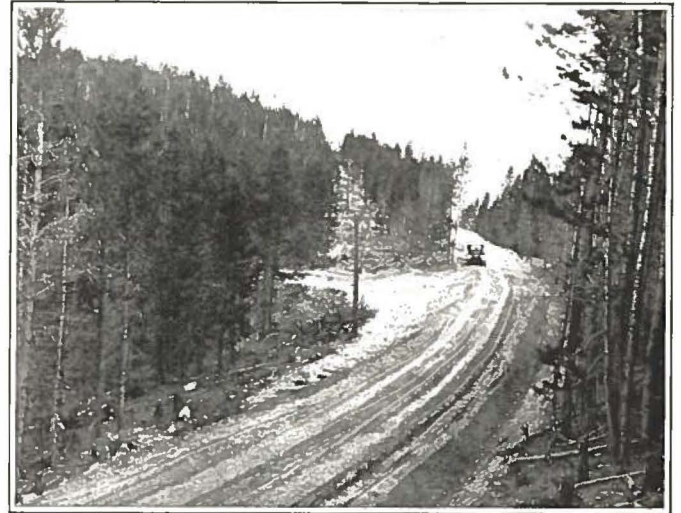
Scene showing completed road and ditches.
