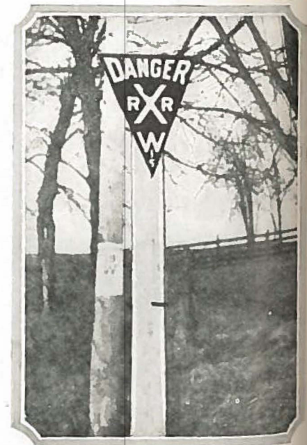
Fig. 3. The standard danger sign for railroad crossings, dangerous hills or curves. (C. 407.)
