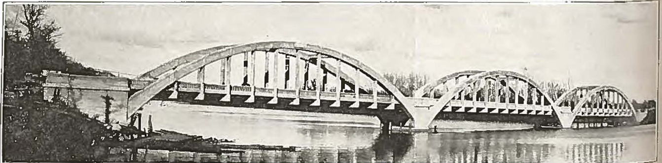
Marsh Rainbow Arch Bridge. This type of bridge will be constructed over the Platte River, at Ft. Morgan, Colo. 1190-foot spans; total length 1060 feet; longest bridge in the state.
